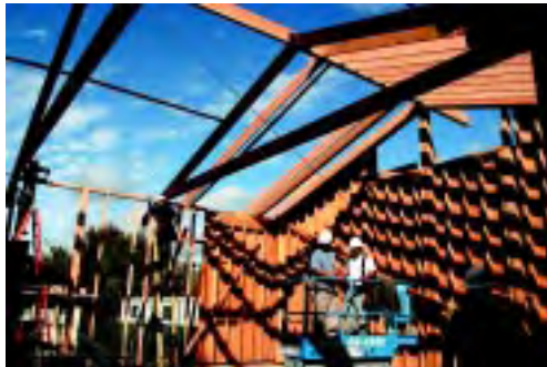
Trusses being framed for new council chambers.
