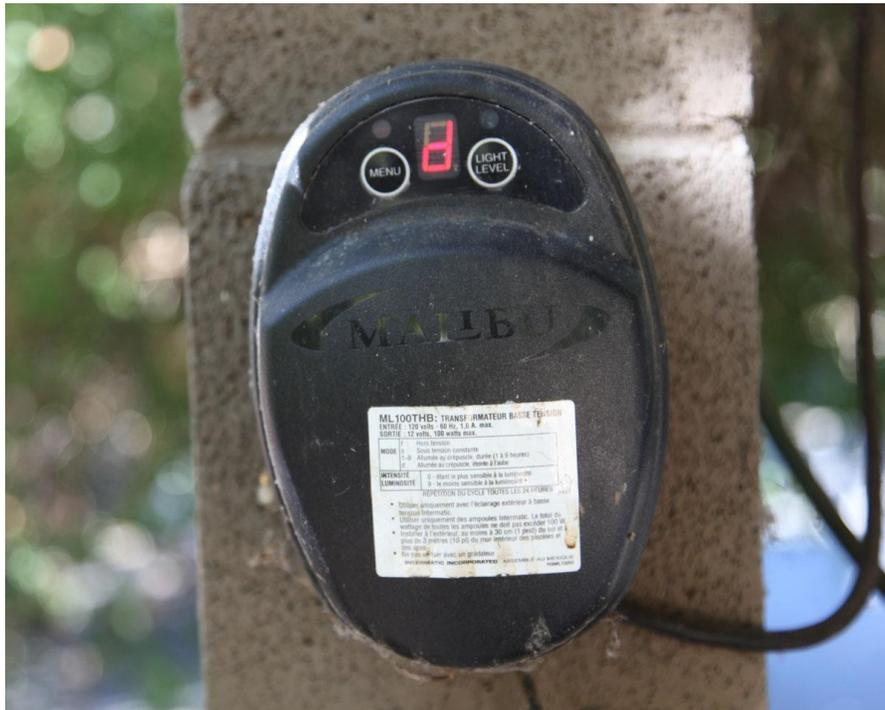
If you are going to use a transformer of the type I used, **CAUTION you have to mount it out of the rain**, but nevertheless somewhere where it receives a lot of daylight - otherwise it won't "see" enough light to cause it to switch off the power to the spotlights. I have mine mounted on a pillar of the car-port - so under the protection of the roof but with a clear view of the sky. And of course you need a 110 volt outlet to plug it into.
